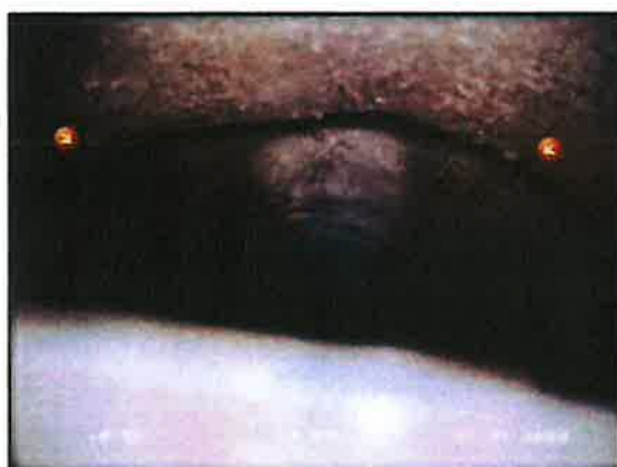
Photo: 7_7_20_A.JPG 21,2m, Fissure circulaire
