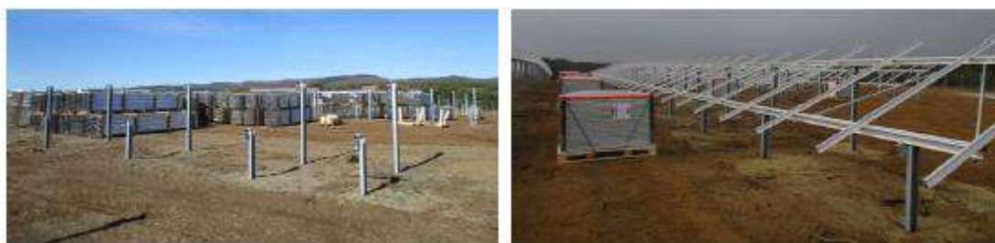
Figure 20 – Photographies de la pose des supports
