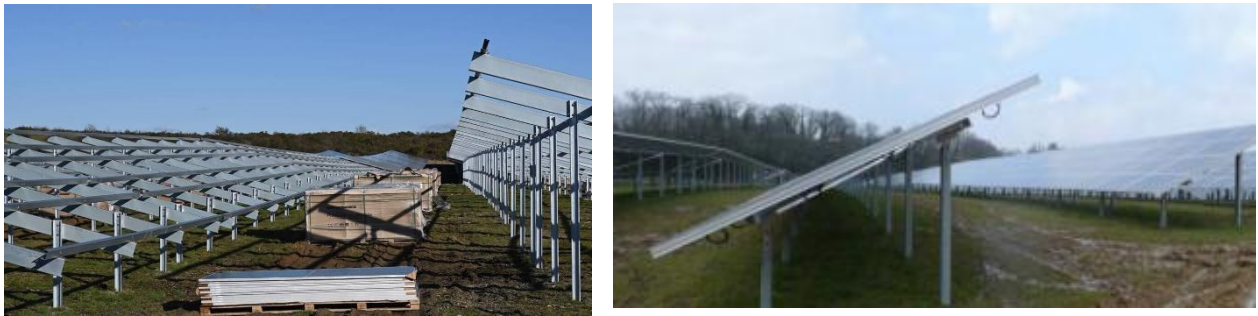
Figure 6: Implantation de pieux battus
