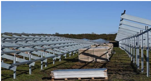
Figure 5: Implantation de pieux battus
