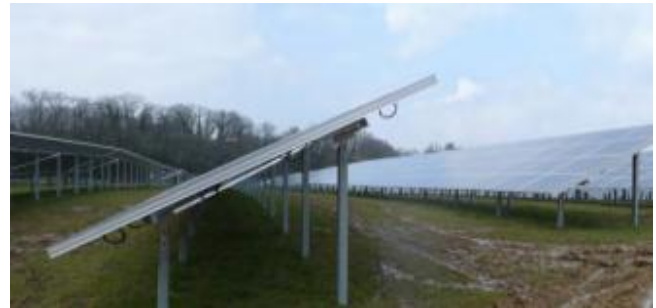
Figure 5: Implantation de pieux battus
