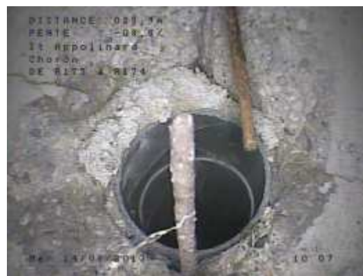
Armatures visibles (CHORON)
