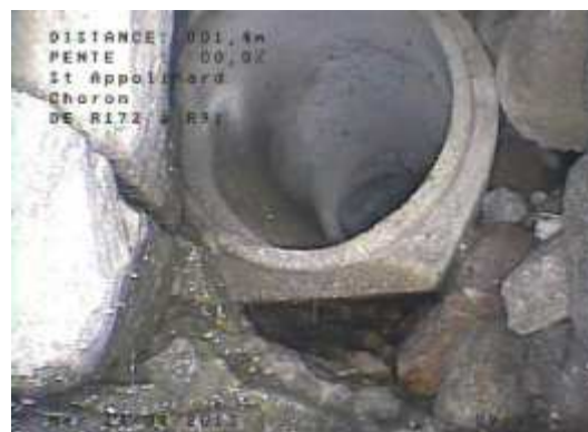
Rupture, Effondrement (CHORON)
