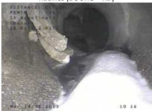
Rupture, Effondrement (CHORON)
