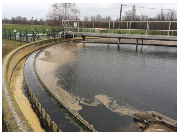
Figure 22 : Clarificateur (1)
