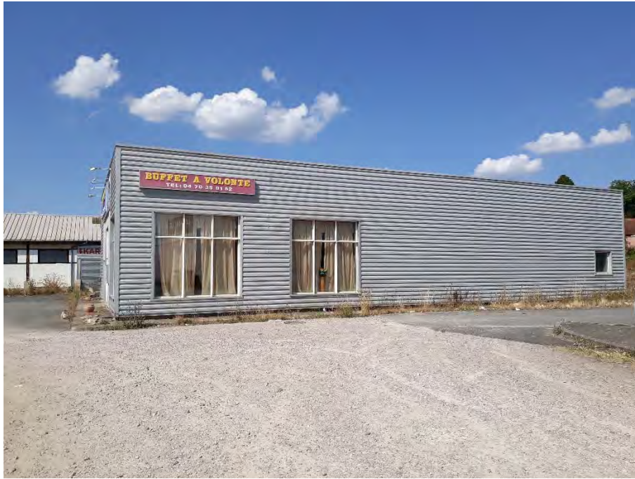
RESTAURANT ASIATIQUE FACADE SUD
