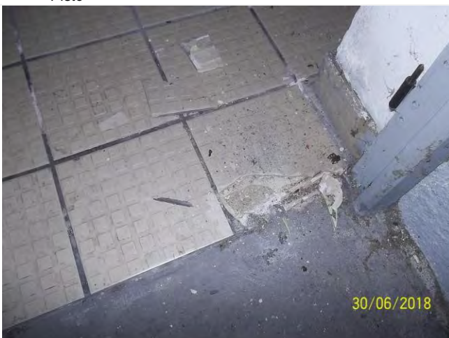
Composant : Colle 39 (N) P16-AR-18-LE-079791-01 RAGREAGE Carrelage 20x20 WC HAND
