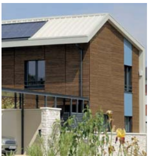
> Maisons passives Atelier Thierry Roche, Saint priest
