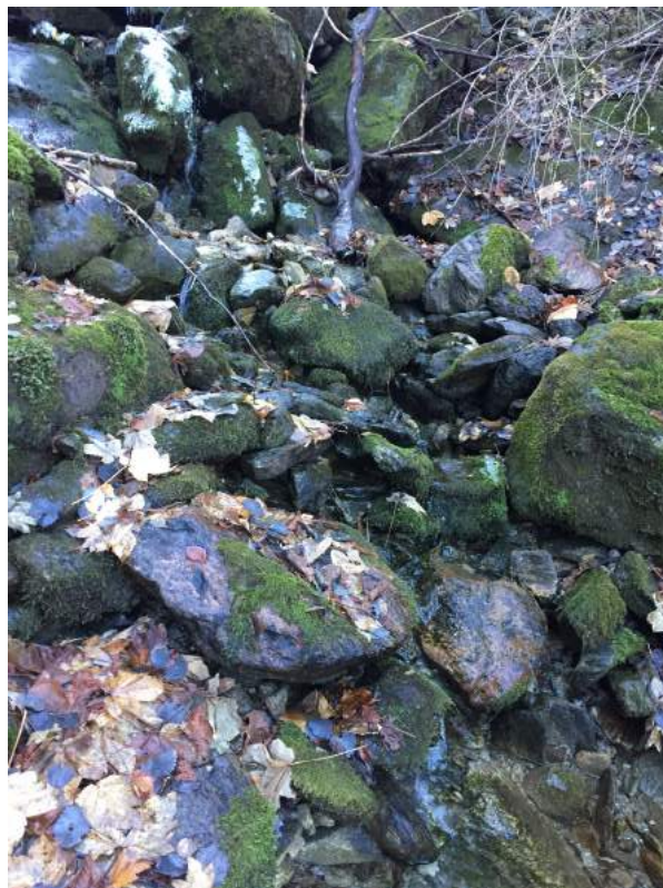
Zone infiltrations Alt 760m
