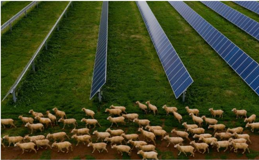
The Blind Creek Solar Farm project, also in NSW, is also using an agrivoltaics model.
