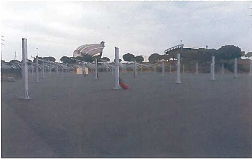
Pose des structures
