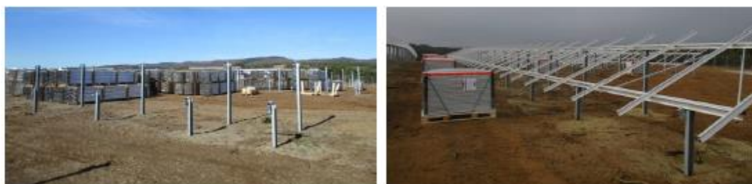
Figure 20 – Photographies de la pose des supports
