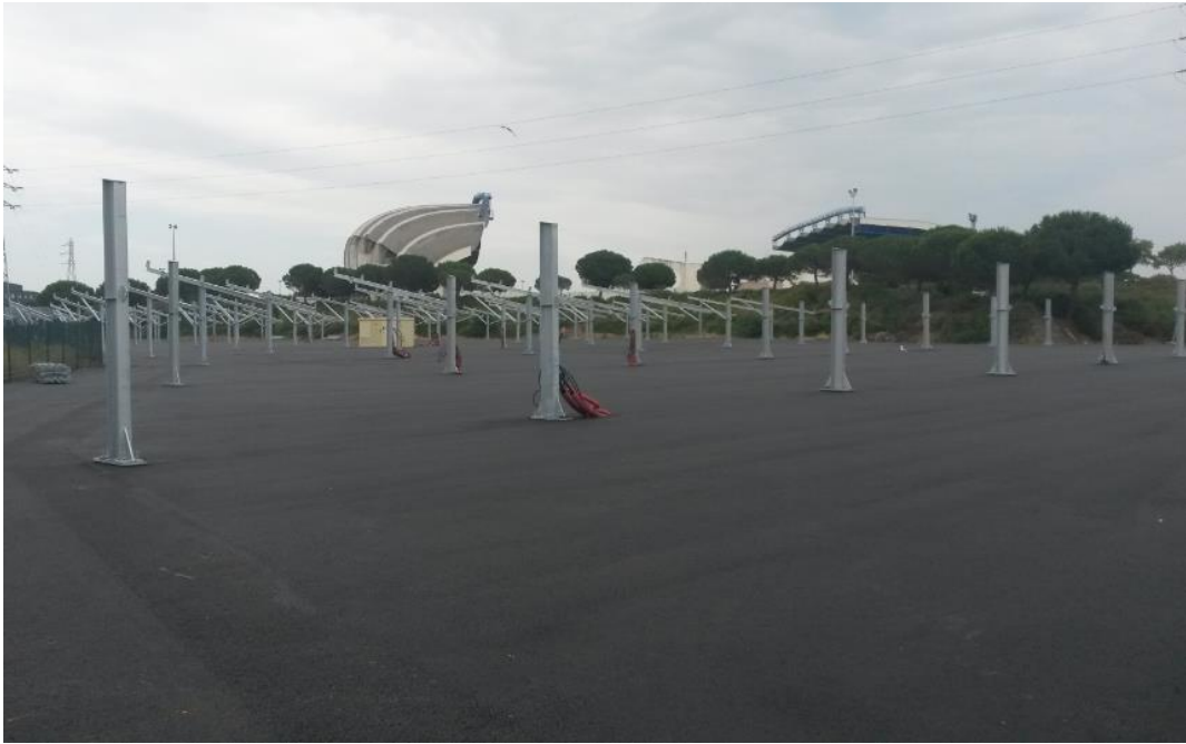
Pose des structures
